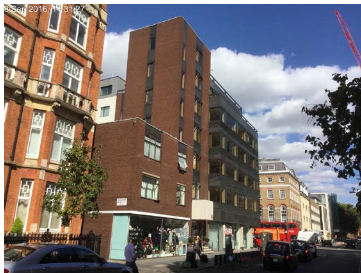
Photograph looking north-west from the south side of Crawford Street.
